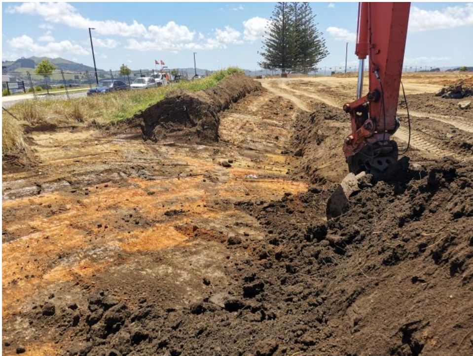
12D fill/toe key area:
