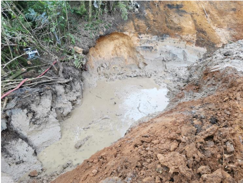
Damaged underfill drain in REB2:
